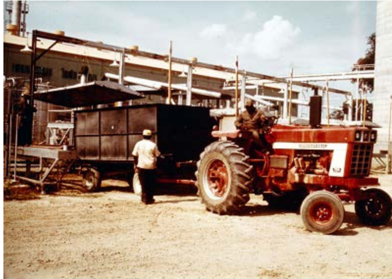
Delivering Truck to the Distillation Unit
