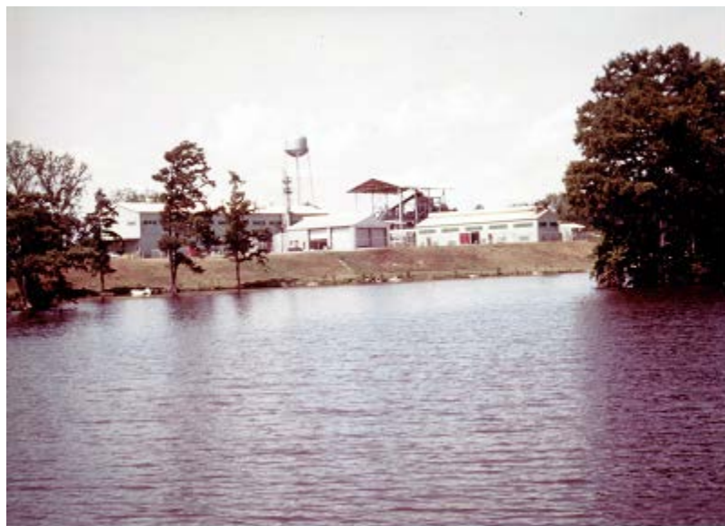
View of Facility from Albemarle Sound
